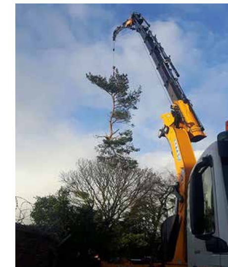
FELLING OPERATIONS WILL BE MORE COMPLEX AND COSTLY THAN USUAL
